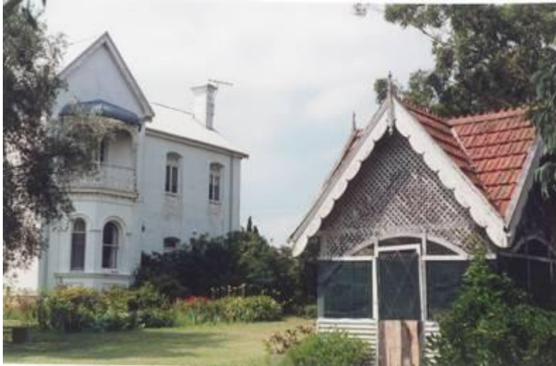
'Upjohn House' and cottage, 1993, Parramatta Heritage Study: Inventory Photo No-335
