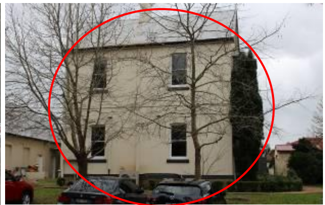
Figure 10: Subject building – viewed from carpark looking at west elevation
