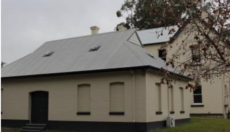
Figure 18a: Rear north facade and recent annex.
