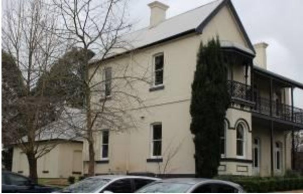
Figure 12: Subject building - West corner
