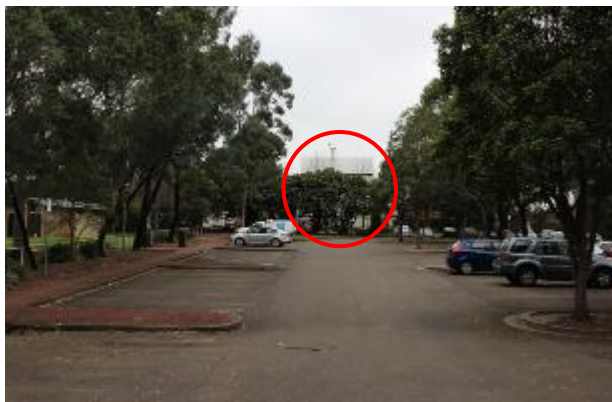
Figure 9: Subject building – viewed from adjacent council owned 'Upjohn Park' carpark, looking at west elevation
